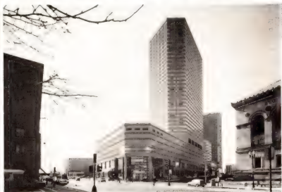
One of the development's hotel towers looms over the public library on Copley Square, right. Mending a hole in the urban fabric, but far from entirely avoiding the fortress syndrome.
